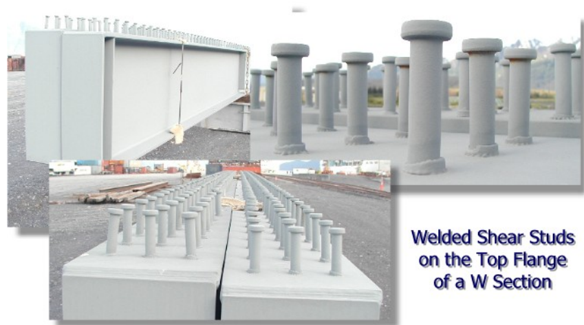
Figure 10.2.2 Typical Welded Studs
