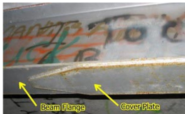
Figure 8.6.2.1 Beam with Cover Plates
