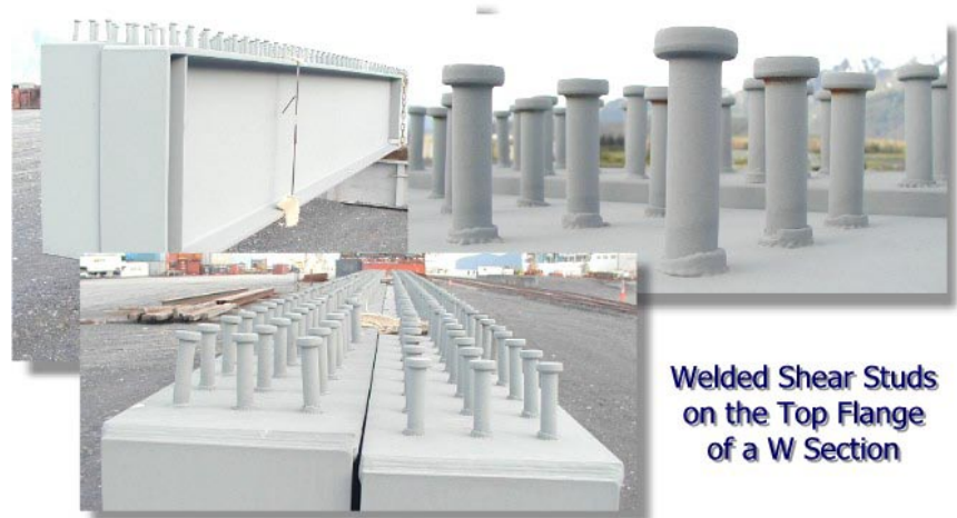
Figure 10.2.2 Typical Welded Studs
